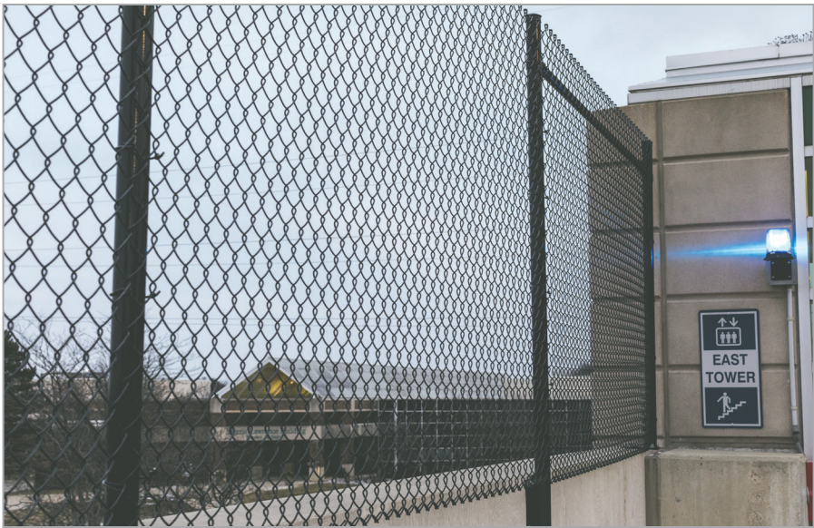
Fencing was installed to the top floor of the campus parking structure as a suicide deterrent.
