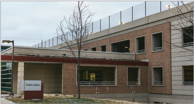
Recently installed fencing to top deck of the campus parking structure is a suicide deterrent measure.
